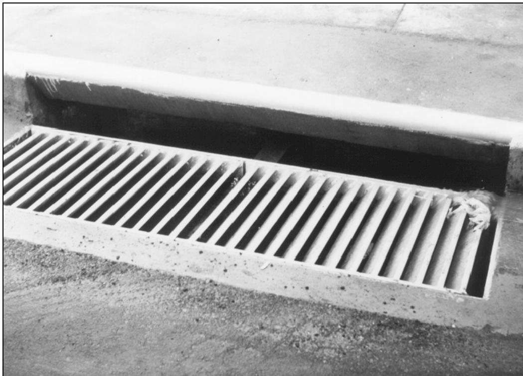
Figure 4-15. Combination curb-opening, 45 degree tilt-bar grate inlet.
