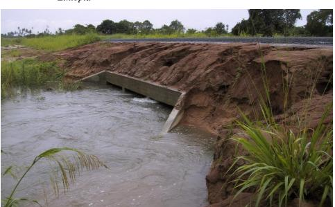
*Figure 4-8 Road shoulder erosion caused from overtopping culvert, Tanzania Ethiopia*
