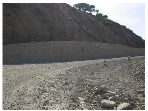
*Figure 4-15* Rockfall protection retaining wall Mekele-Abi Adi-Adwa km 52+3, Ethiopia
