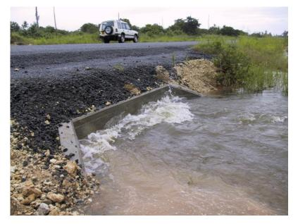
*Figure 6.1 Example of inadequate culvert sizing when climate changes*
