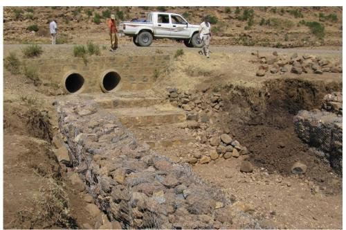
Figure 4-9 Increased culvert outlet protection Mekele-Adwa km 68+722, Ethiopia
