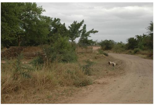
Figure 5.1 Bridge in Mozambique partly washed away
