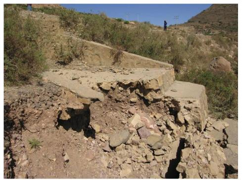
Figure 4-6 Eroded culvert outlet protection Mekele-Adwa km 39+038, Ethiopia
