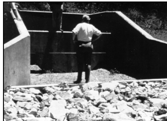
Figure 10.3b. Baffle-wall energy dissipator, USBR Type VI.
