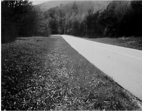
Figure 5.2. Vegetative channel lining.
