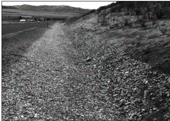
Figure 5.3. Riprap channel lining.
