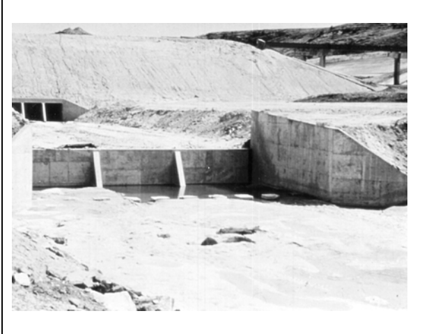
Figure 10.4. Straight drop spillway stilling basin.
