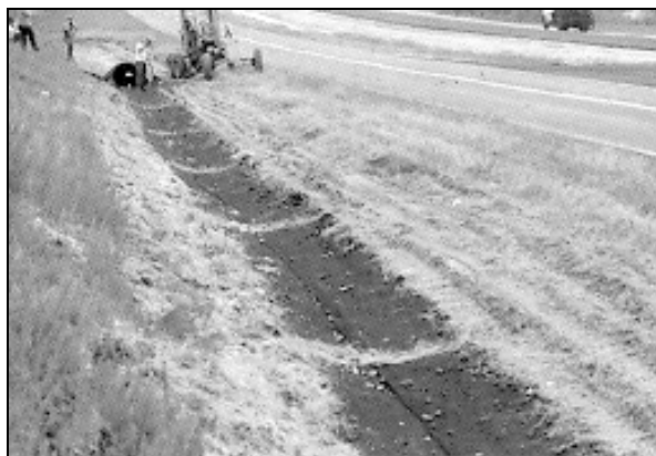
Figure 5.5. Installed TRM channel lining.
