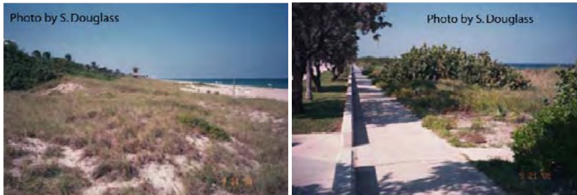
Figure 7.16. Beach nourishment project with constructed dune on top of old, failed revetment protecting road. Florida Highway A1A, Delray Beach (2001)
