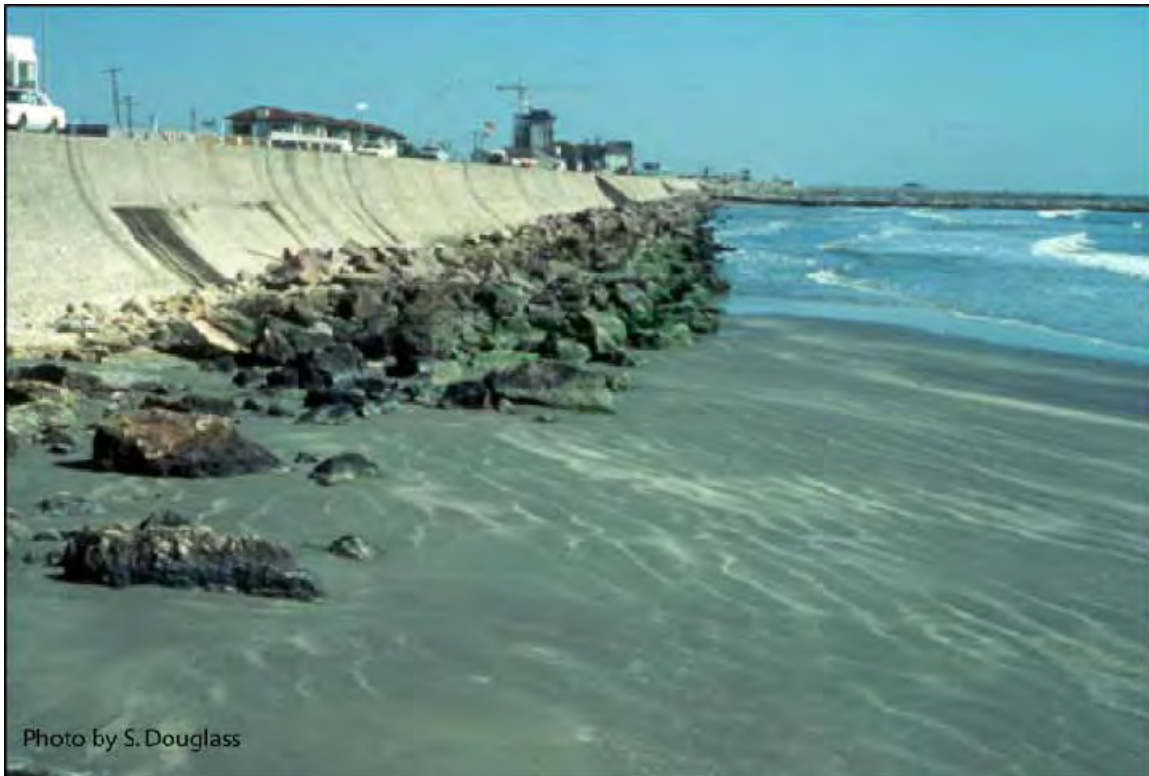
Figure 6.3. Galveston Seawall. Seawall Boulevard (1983)
