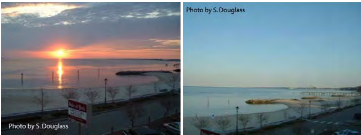
Figure 7.24. Beach nourishment project stabilized as pocket beaches with a headland breakwater system protecting a road (Water Street, Yorktown, Virginia)
