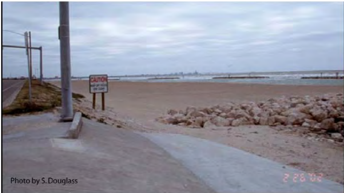
Figure 7.22. Offshore segmented breakwaters with groins and beach nourishment on Corpus Christi Bay (Ocean Drive, Corpus Christi, Texas).
