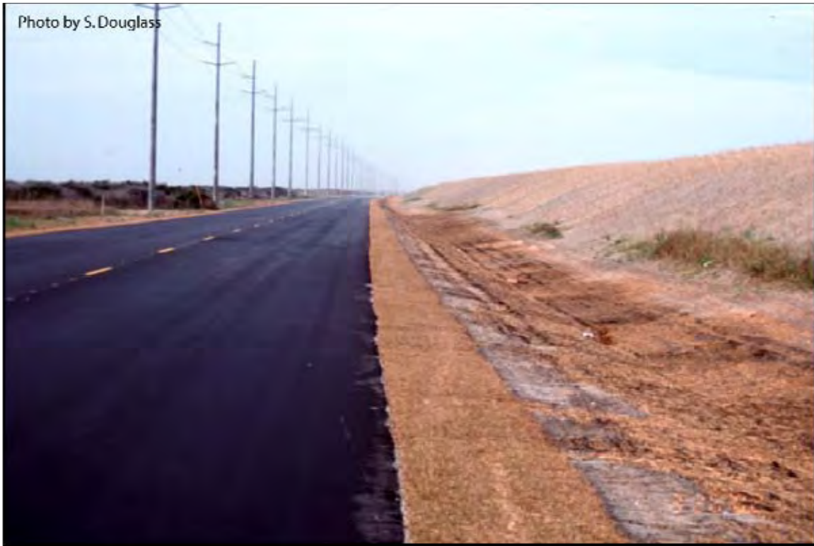
Figure 8.18. Artificial sand dune constructed seaward of a highway to protect the highway (North Carolina Highway 12)
