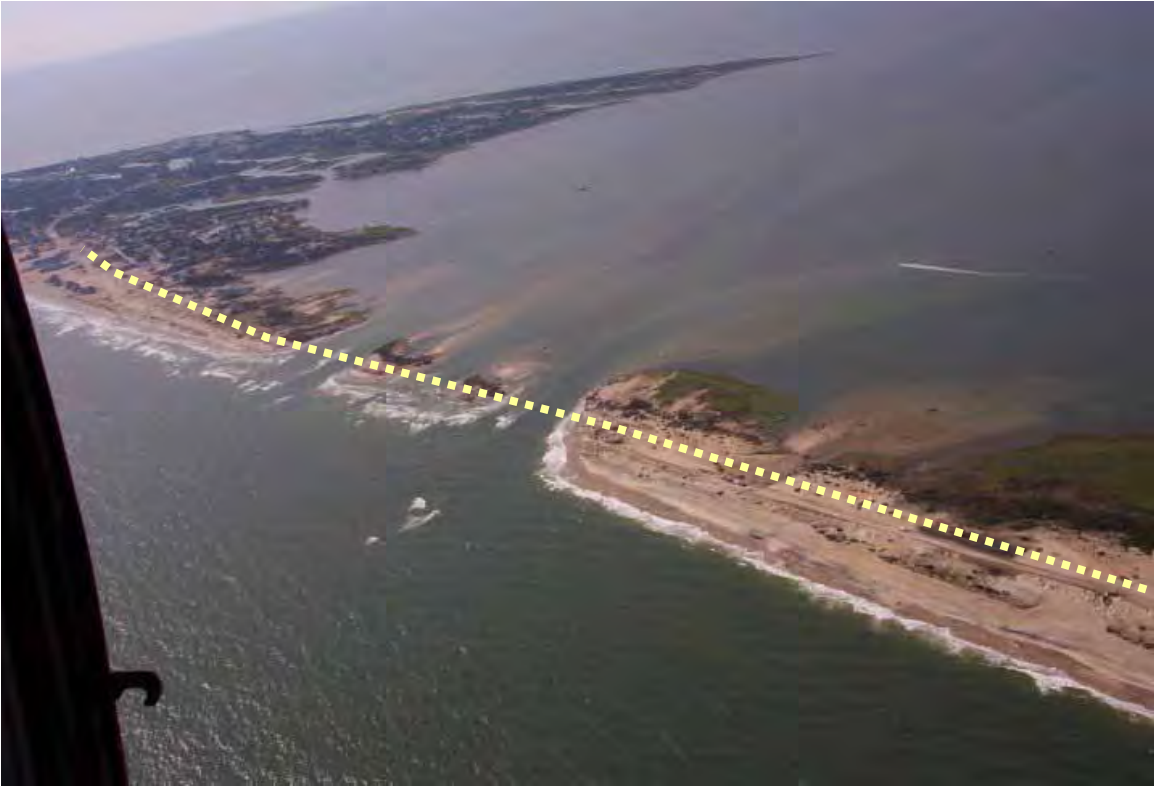
Figure 2.6. Breaches in Outer Bank barrier island caused by Hurricane Isabel in 2002 (NC 12 ROW is dotted line).
