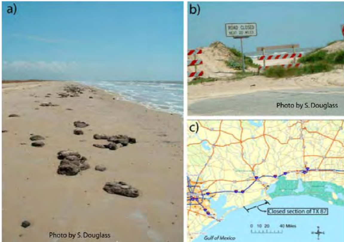
Figure 7.5. Road destroyed by shoreline recession: a) broken pavement on the beach at the old location; b) south end of the closed section; c) location map. Texas Highway 87, Jefferson County (2002)
