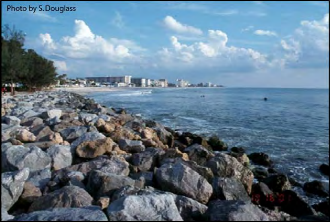
Figure 6.5. Seawall protecting a coastal highway. Venice, Florida (2001)
