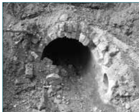
Figure 8.12 The culvert during demolition (courtesy Andy Pepper)
