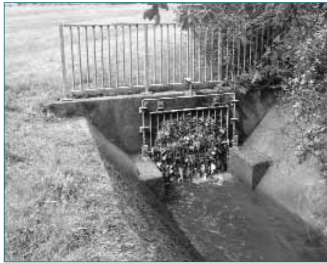
Figure 9.28 Security screen blocked from the inside (courtesy Andy Pepper)
