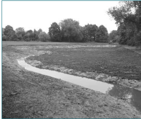
Figure A3.38 As-constructed re-alignment of watercourse post-daylighting (courtesy Andy Pepper)
