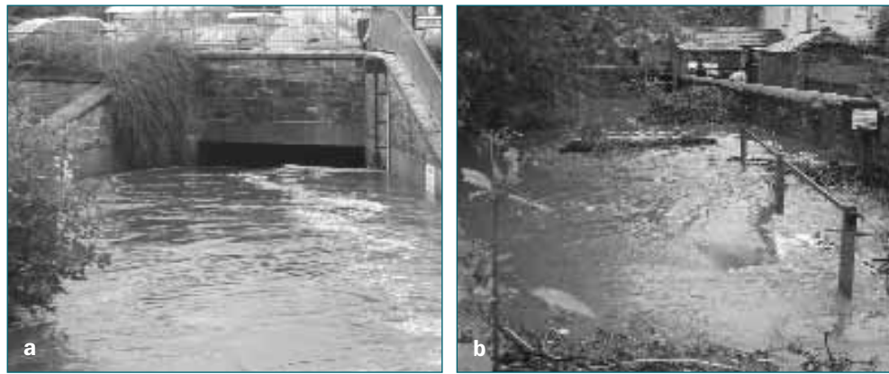
Figure 6.9 Free (a) and submerged (b) flow during flood conditions (courtesy JBA Consulting)
