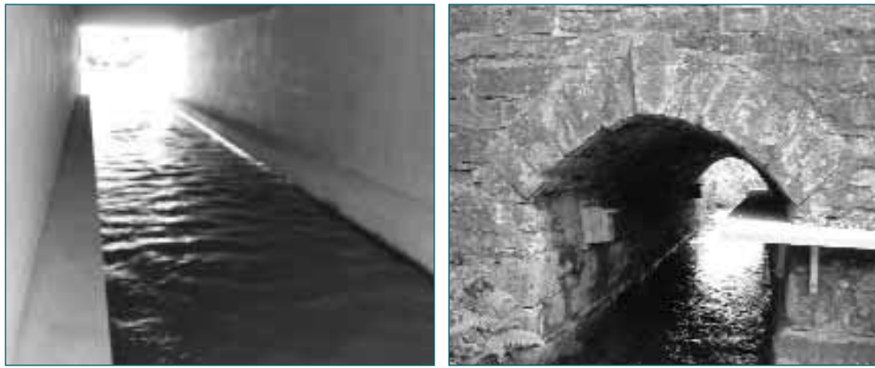
Two approaches to the provision of access through a culvert for mammals. On the left a new concrete culvert has built-in ledges on both sides. On the right a steel ledge has been retrofitted to an old culvert (note also nesting boxes). In both cases it is necessary to consider the level of the ledge with respect to normal and floodwater levels and its effect on debris passage and hydraulic performance. An alternative approach is to provide a dry passage parallel to the culvert (see Figure 9.24). See also Case study A3.5.
