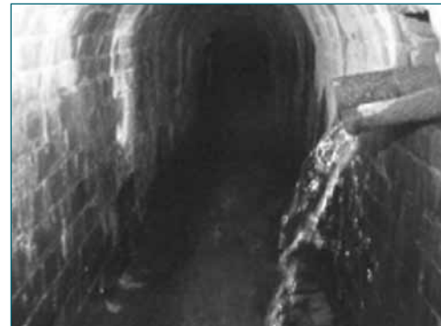
Figure A3.25 Inside the culvert, showing a peculiar drainage inflow
