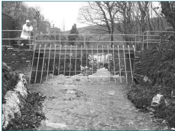
Figure A3.40 River Jordan debris screen as-built (courtesy Environment Agency)
