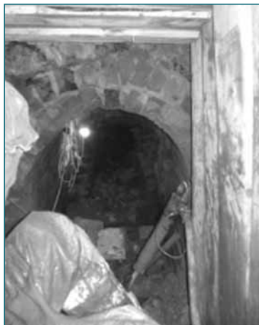
Figure A3.28 Installation of new timber framed heading
