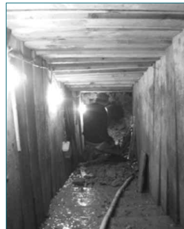
Figure A3.29 Installation of new timber-framed heading
