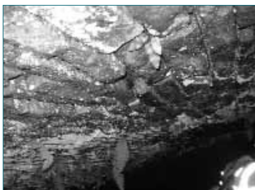
Figure 8.4 Typical large masonry culvert showing general mortar loss to the culvert barrel (courtesy Ferro Monk)
