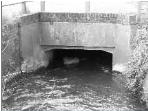
Figure 6.19 Culvert flowing under inlet control
