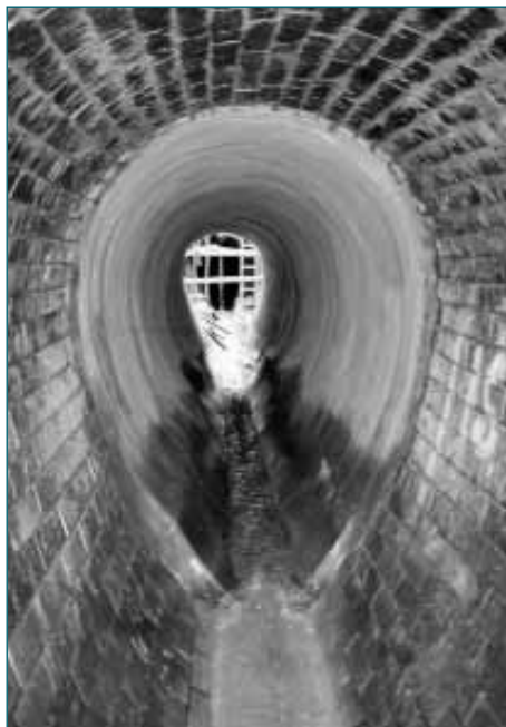
Figure 8.7 Sprayed lining to a masonry culvert (courtesy Ferro Monk)
