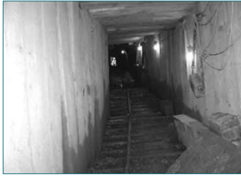
View showing completed timber-framed heading
