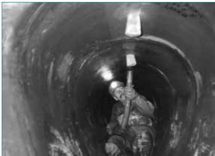
Figure 8.8 Grouting of GRC liner (courtesy Ferro Monk)
