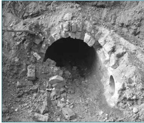
Figure A3.36 Demolition of brick-lined culvert (courtesy Andy Pepper)
