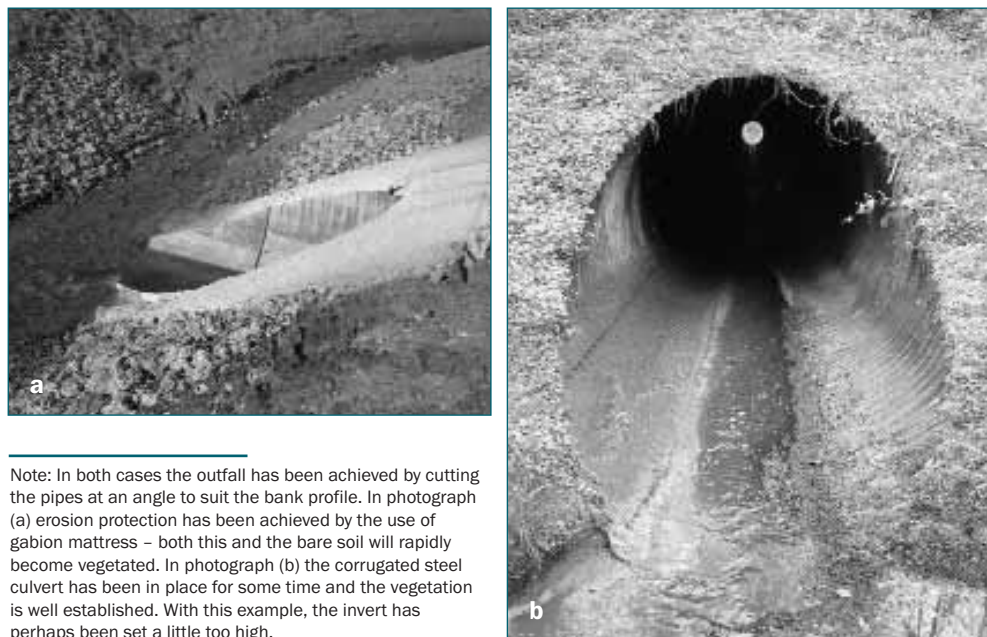
Figure 9.29 Two simple outfall structures: concrete pipe (a) and steel pipe (b) (courtesy Andy Pepper and Amanda Kitchen)
