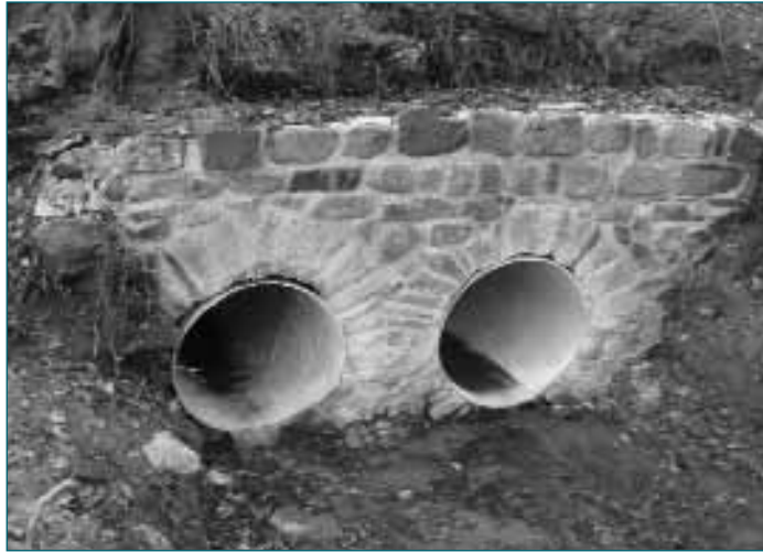
Figure 8.6 Slip lining of a masonry culvert (courtesy British Waterways)
