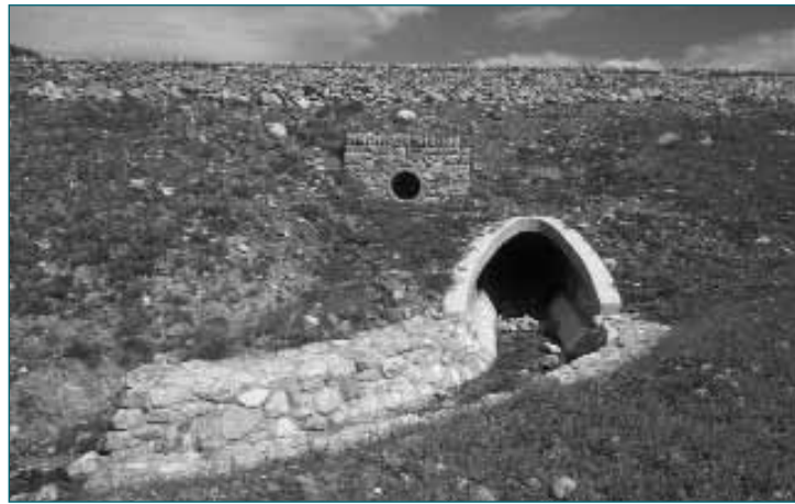
Note the simple outlet arrangement, with mortared stone pitching channel lining on the bend in the watercourse. Note also the gravel invert in the culvert (matching that in the watercourse), the use of local stone, and provision of a mammal crossing at higher level.
