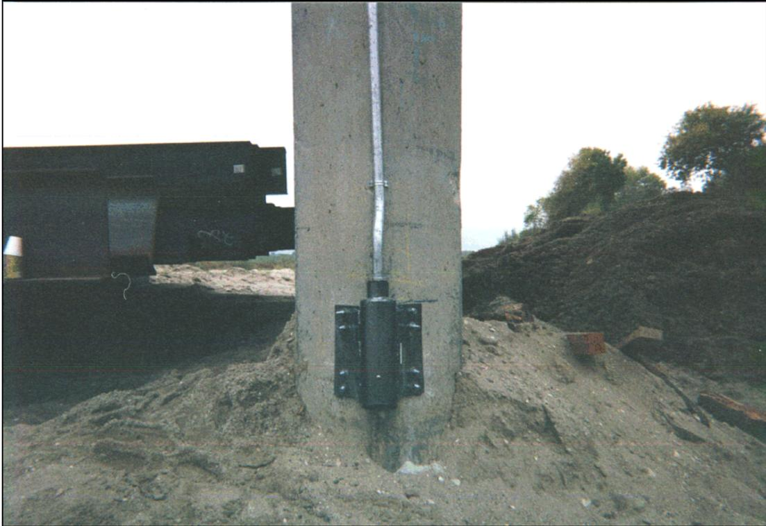
Figure 9.28. Close up of sonar scour monitor on Salinas River Bridge near Soledad, CA.
