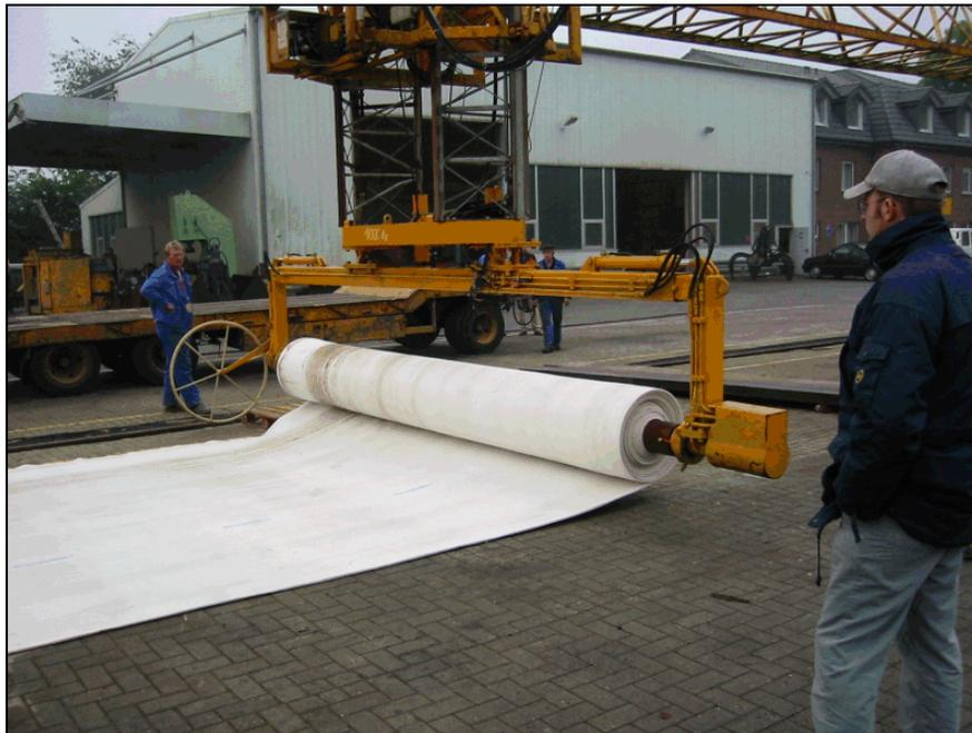
Figure 5.3. SandMat™ geocomposite blanket being unrolled.
