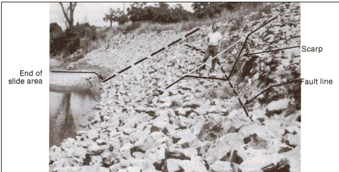
Figure 5.11. Riprap on Cosumnes River at Site 2 near Sloughouse, CA, looking downstream, showing translational slide failure (photographed May 31, 1983) (Blodgett & McConaughy 1986).
