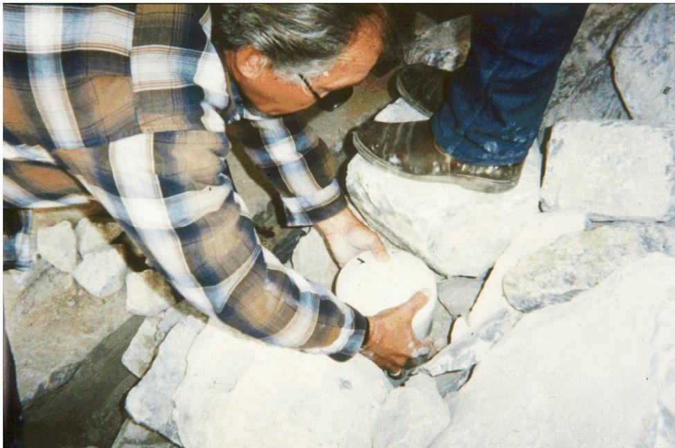
Figure 9.32. Installation of a float out device by Nevada DOT to monitor riprap stability.
