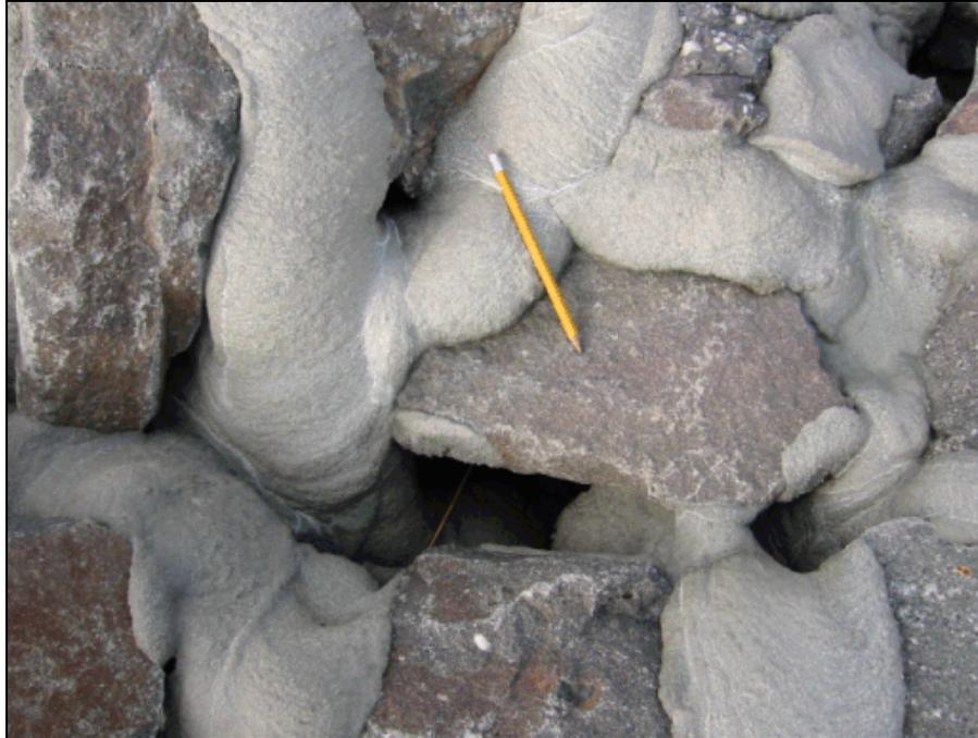
Figure 5.20. Close-up view of partially grouted riprap.
