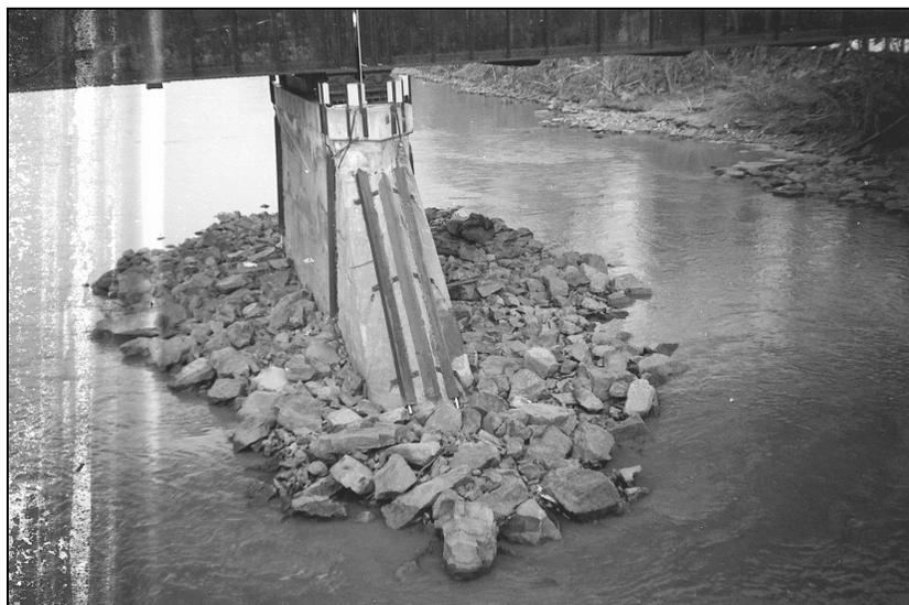
Figure 9.21. Brisco Monitor sounding rods installed at a bridge pier in New York to monitor movement of riprap (Butch 1996).
