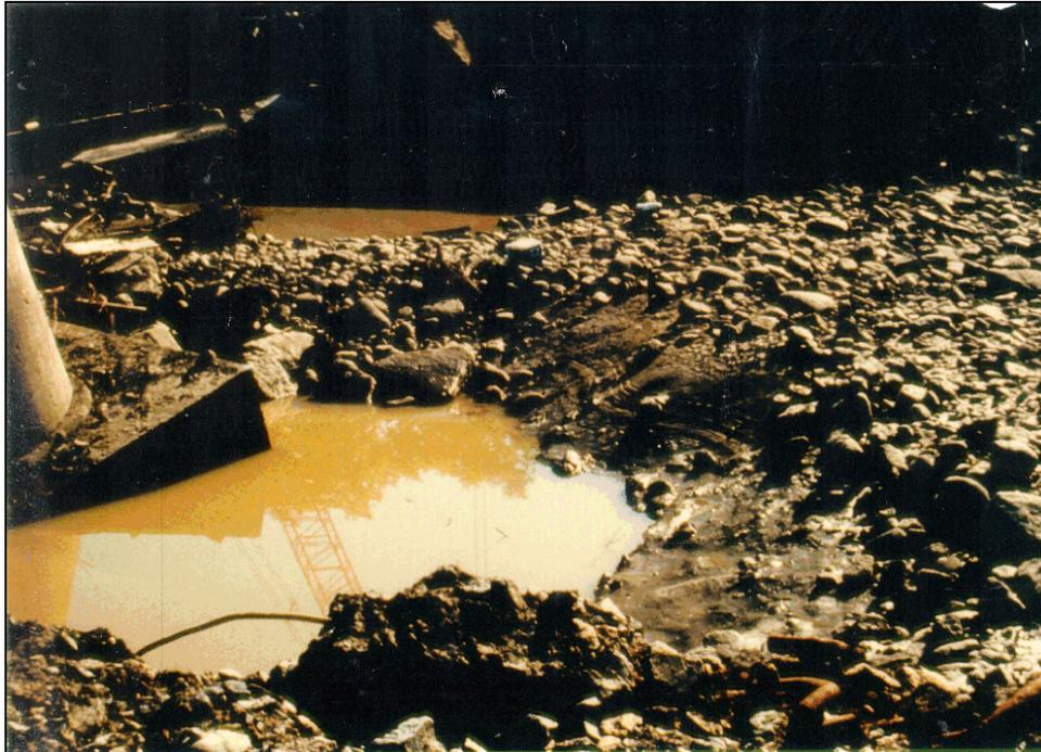
Figure 5.17. Pier scour holes at Schoharie Creek Bridge in 1987. Pier 2 in the foreground with pier 3 in the background.
