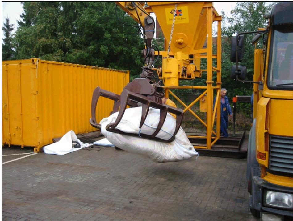
Figure 5.6. Handling a 1.0 metric tonne sand-filled geotextile container.
