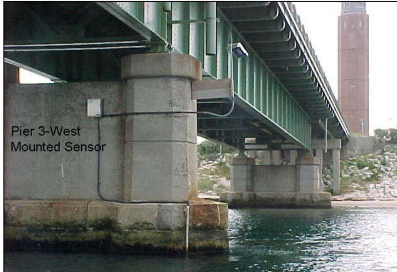
Figure 9.13. Sonar scour monitor installation including remote station and solar panel.
