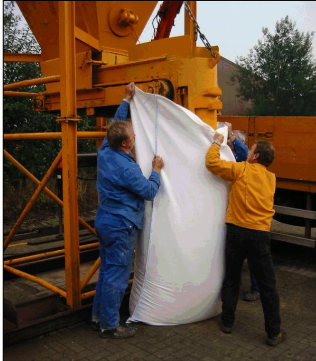
Figure 5.5. Filling 1.0 metric tonne geotextile container with sand.
