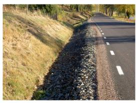
Fig.1. Surface drainage system, photo: VTI
