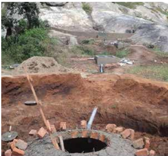
Borehole for rainwater harvesting in Uganda
