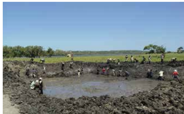
Digging of fish pond.
