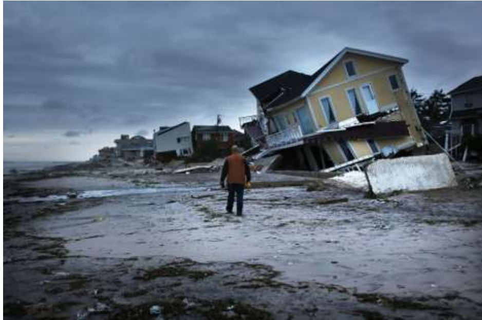
Damage in the Rockaway neighbourhood of Queens, New York, where the boardwalk was washed away during Hurricane Sandy in 2012. Photograph: Spencer Platt/Getty Images
