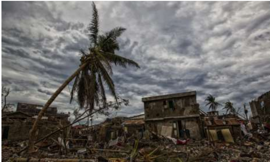
Damage to homes in the town of Jeremie, Haiti, after the arrival of Hurricane Matthew in 2016. Photograph: Logan Abassi/AFP/Getty Images
