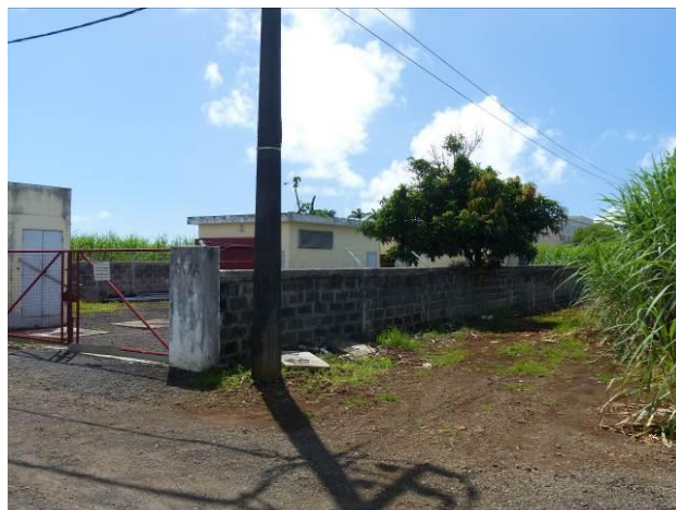
Figure 4-7: CWA Groundwater Pumping Station BH 548
