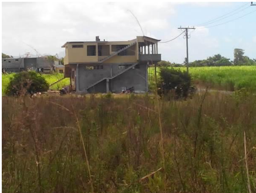
Figure 4-12: Detached house under construction immediately next to the proposed roundabout on La Barraque Road (part of agglomeration belonging to Plaine Magnien)
