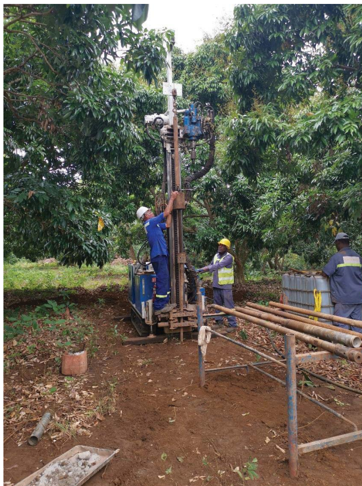
Figure 3. 3: Drilling work at PBH 2
