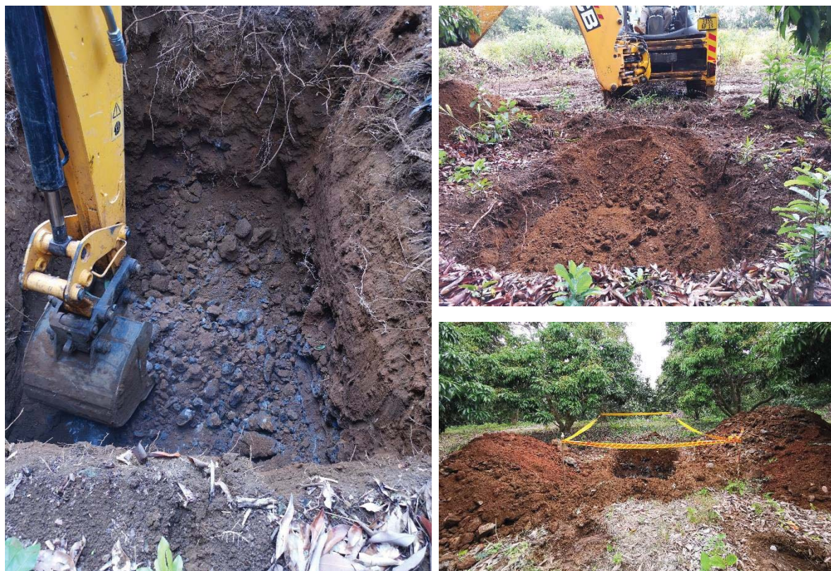
Figure 3. 2: Trial pit investigations
