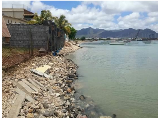
Dumped mass concrete and rock
