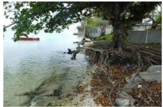
Existing Site Waterfront to NW
