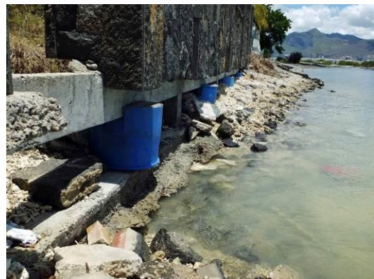
Underpinned wall
