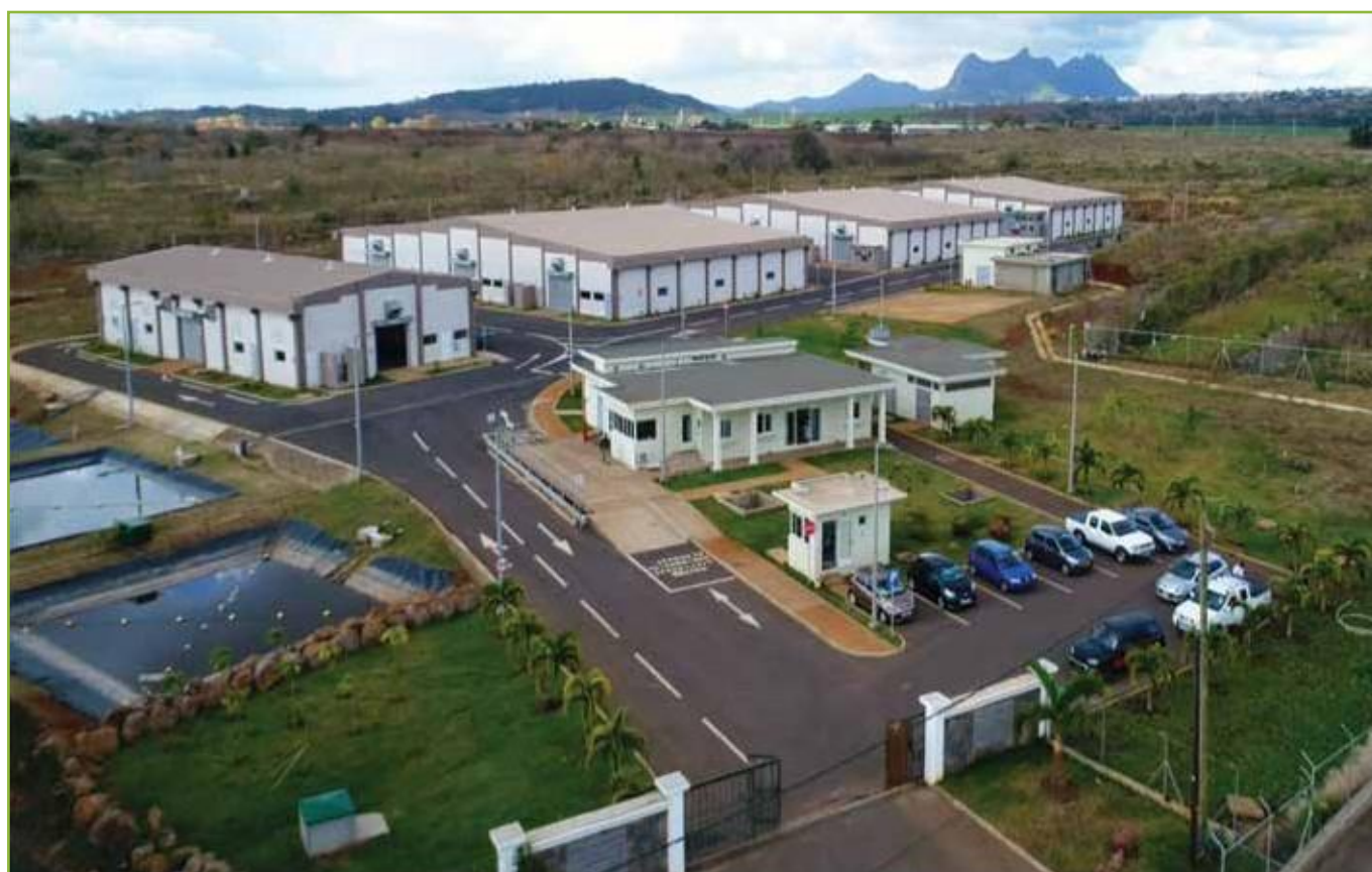
Figure 16: Interim Storage Facility for Hazardous Wastes
