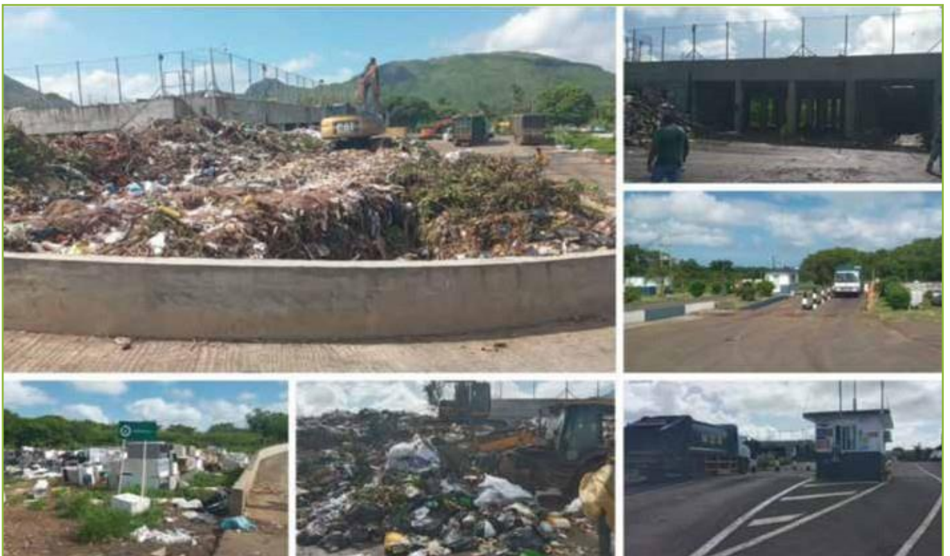
Figure 13: La Chaumière Transfer Station
