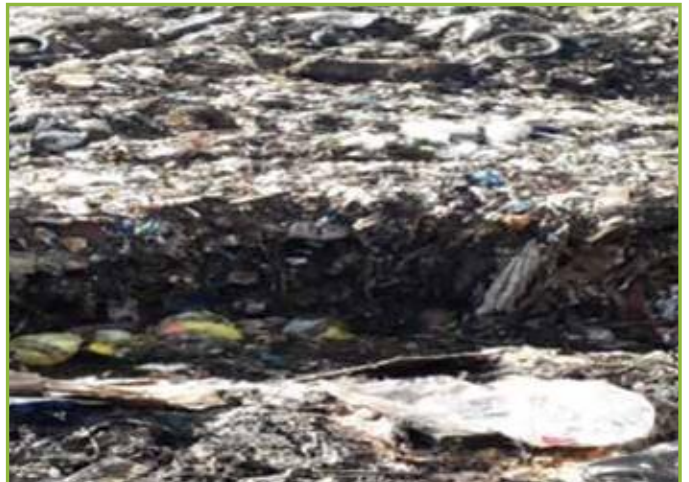
Figure 25: Wrapped asbestos sheets are disposed at Mare Chicose landfill through trenching
