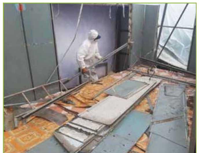
Figure 22: Dismantling of cemented asbestos sheets in enclosed housing unit
