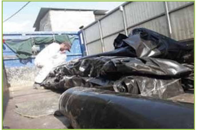
Figure 24: Loading of wrapped Asbestos sheets on lorry for carting away
