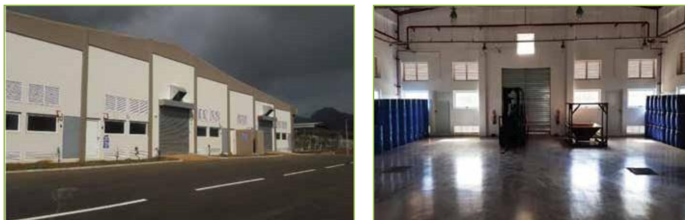
Figure 27: Interim Storage Facility for Hazardous waste at La Chaumiere.
