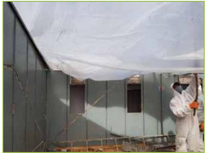
Figure 20: Setting up of enclosure prior to starting the dismantling of asbestos housing unit
