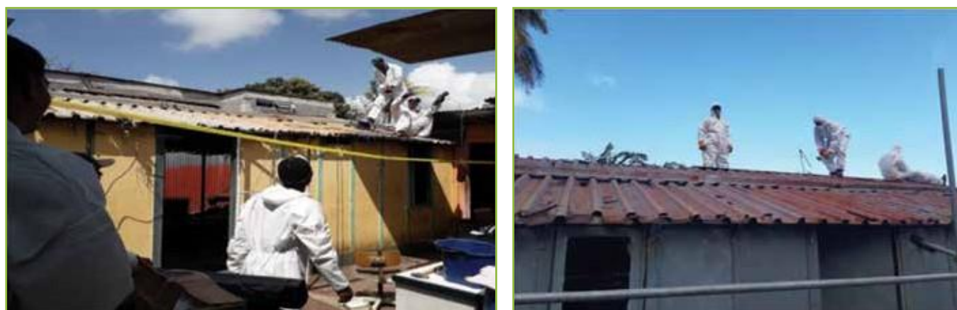
Figure 19: Removal of corrugated sheets from the roof the asbestos housing unit
