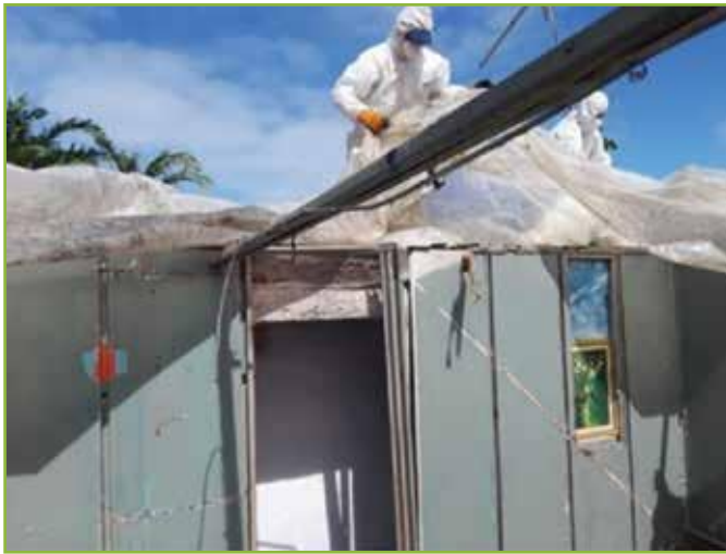
Figure 20: Setting up of enclosure prior to starting the dismantling of asbestos housing unit
