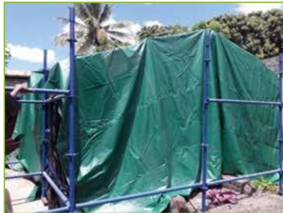
Figure 21: Asbestos housing unit already enclosed and ready to be dismantled
