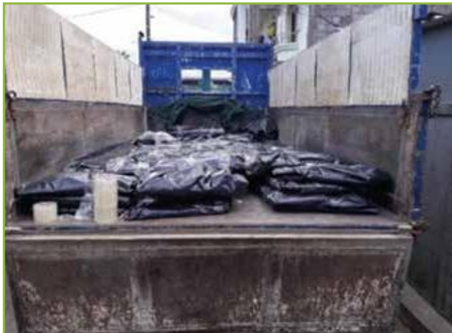
Figure 25: Wrapped asbestos sheets are disposed at Mare Chicose landfill through trenching
