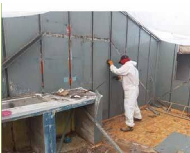
Figure 22: Dismantling of cemented asbestos sheets in enclosed housing unit
