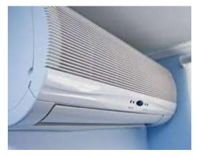
Avoid installing your air-conditioner in direct sunlight which could jeopardize the cooling effect.
