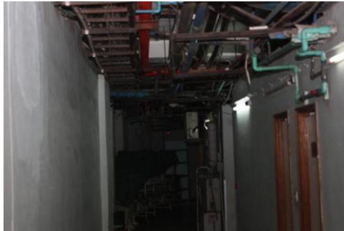
**IGMH – Narrow Corridors, Fire System need rehab and Inadequate Means of Egress (No signs and open doors)**
