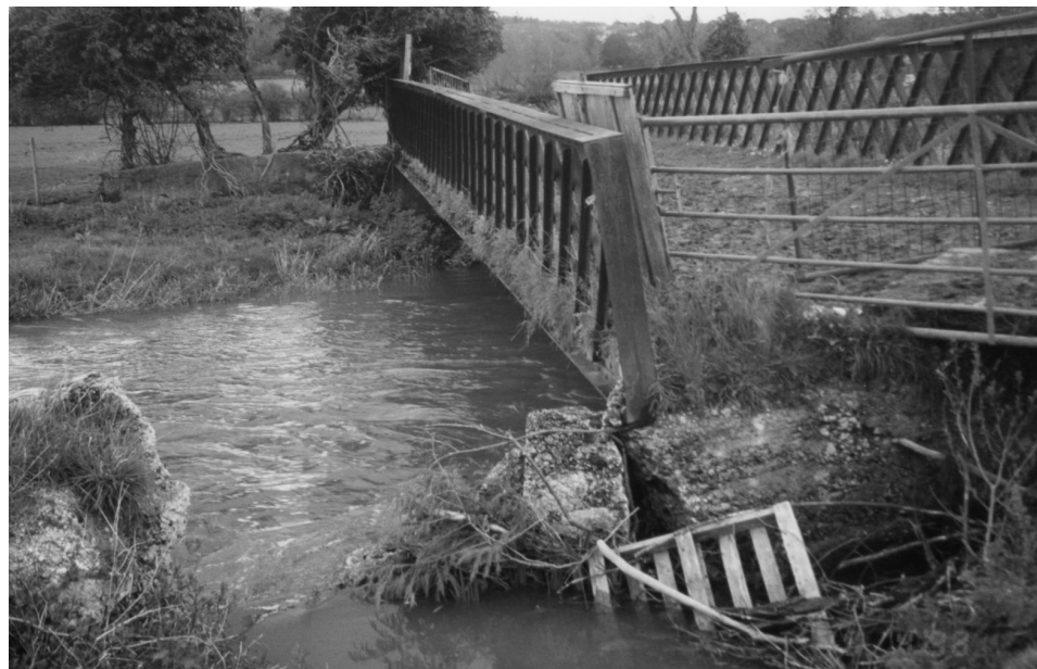
View of right abutment
