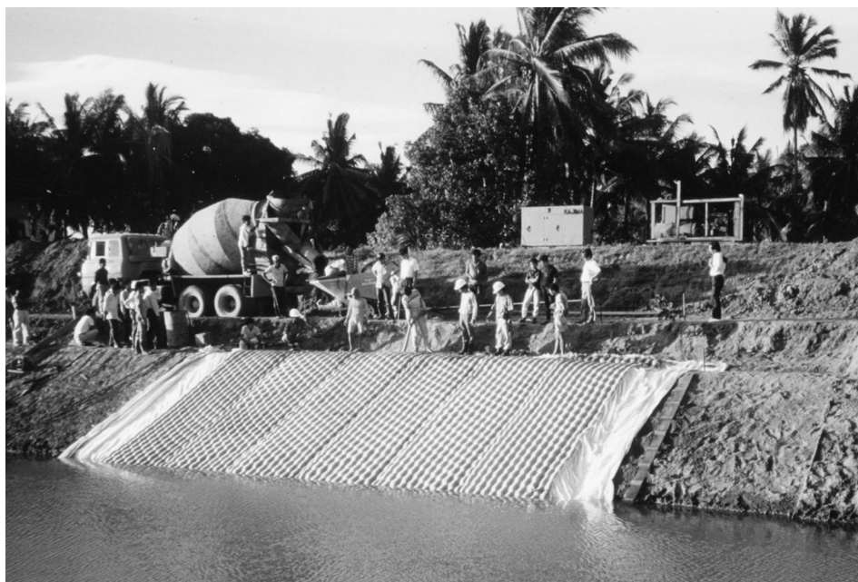
Grout-filled mattress protection to channel bank
