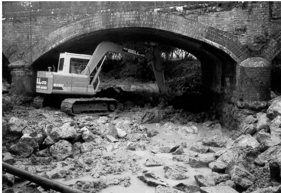
Figure 5.42 Placing riprap in restricted headroom (photograph courtesy of Jeremy Benn Associates)
