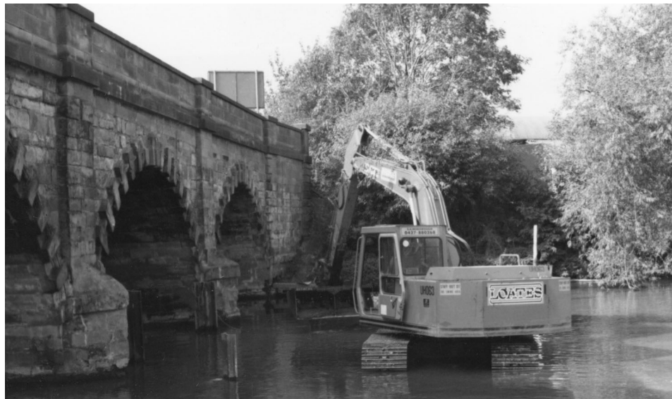
Figure 5.41 Scour protection works being undertaken in ideal conditions
