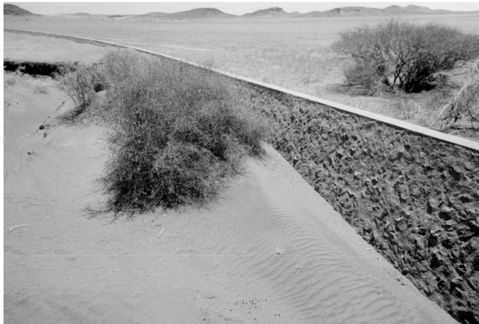
Figure 5.17 Guide wall on approach to a bridge across an alluvial fan. This view is looking upstream from the bridge. The wall channels water flowing from left to right, to avoid outflanking of the bridge
