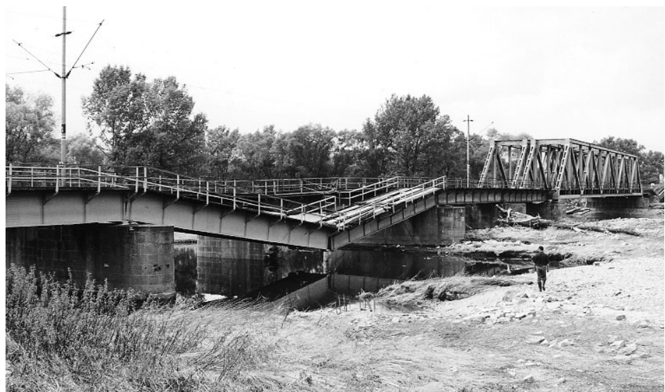
Figure 5.1 Effects of scour damage (photographs courtesy of Czech Railways Infrastructure Division)
