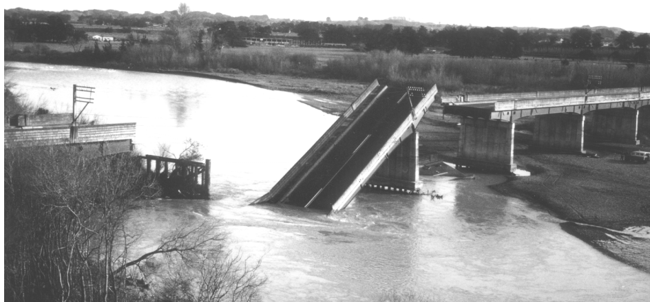
Figure A2.5 Bulls road bridge failure (photograph courtesy of Bruce Melville)
