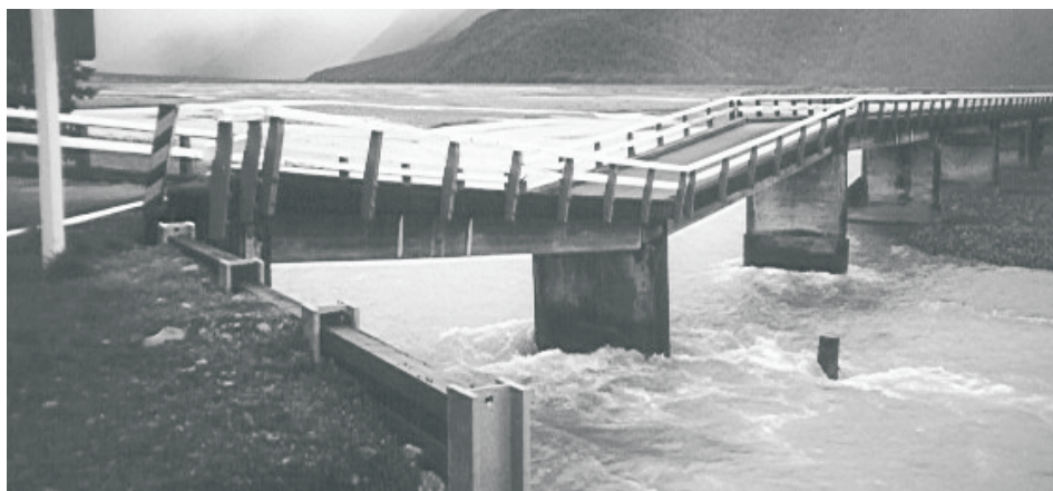
Figure A2.6 Bealey bridge failure (photograph from Coleman et al, 2000, by permission of the authors)
