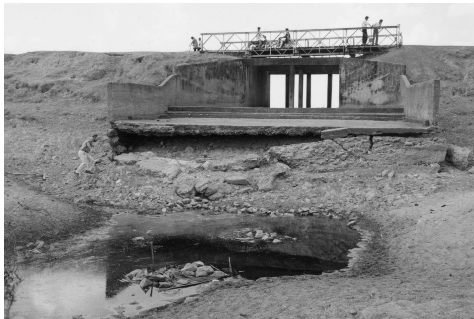
Figure 5.40 Scour downstream of an offtake structure, caused by the lack of scour protection coupled with inadequate energy dissipation
