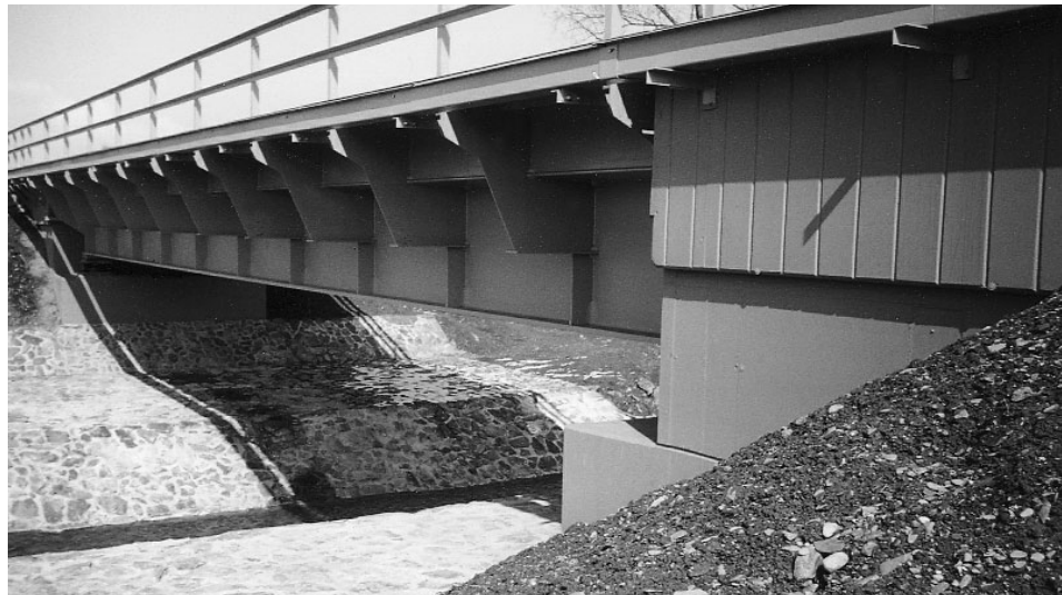
Figure 5.31 Grouted stone pitching to bridge invert (photograph courtesy of Czech Railways Infrastructure Division)
