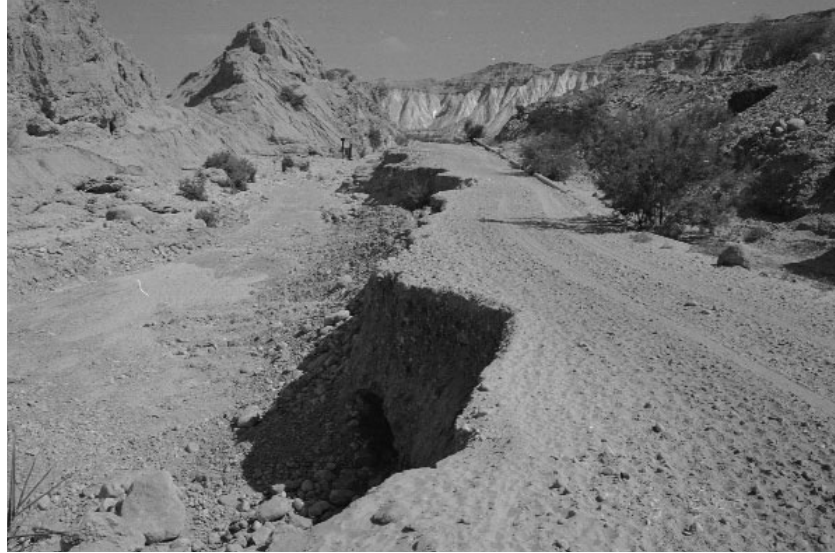
Figure 5.2 Road undermined by lateral erosion from an upland wadi
