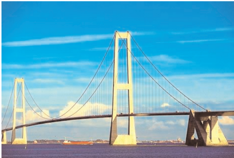
Figure A2.1 The combined road and railway bridge across the western channel of the Storebælt between Fyn and Sprogø (photograph courtesy of Great Belt A/S)
