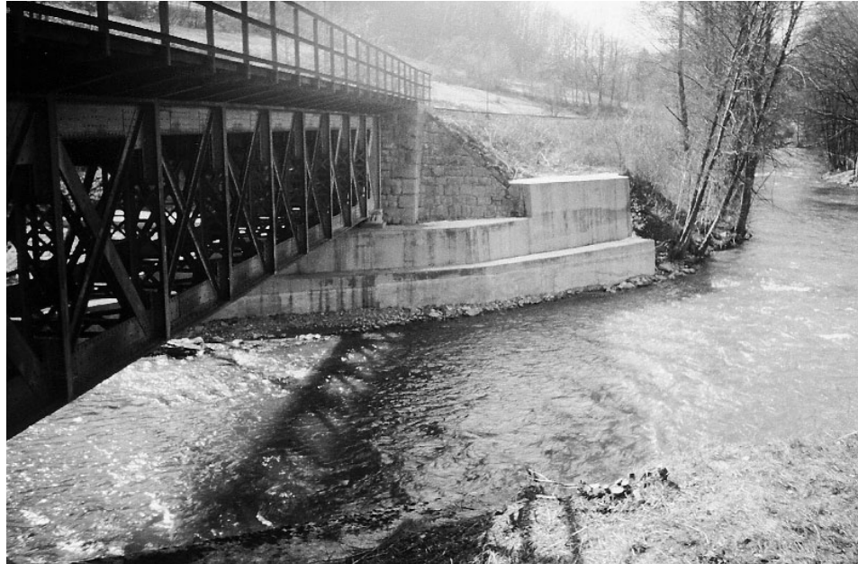
Figure 5.23 Concrete repairs to a bridge abutment (photograph courtesy of Czech Railways Infrastructure Division)
