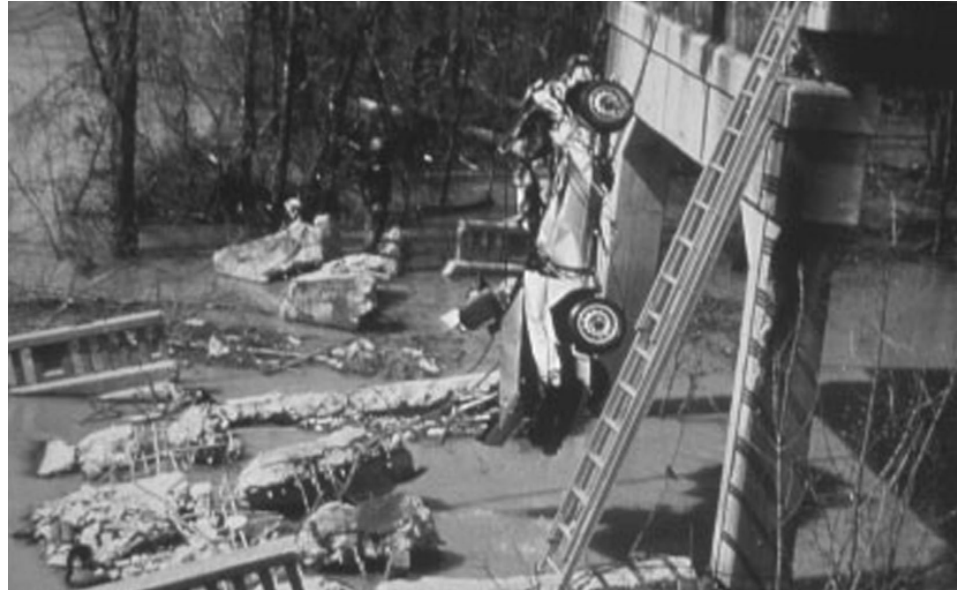
Figure A2.9 The aftermath of the Hatchie River bridge failure (photograph courtesy of Ayres Associates)
