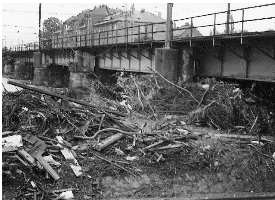
Figure 5.9 Blockage by debris (photograph courtesy of Czech Railways Infrastructure Division)
