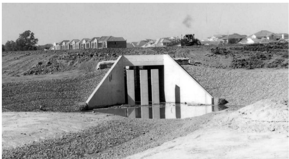
Gabion protection at energy dissipator
