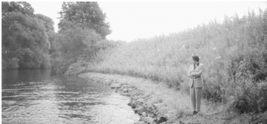
Figure A2.4 The protected embankment six months after construction (photograph courtesy of Jeremy Benn Associates)
