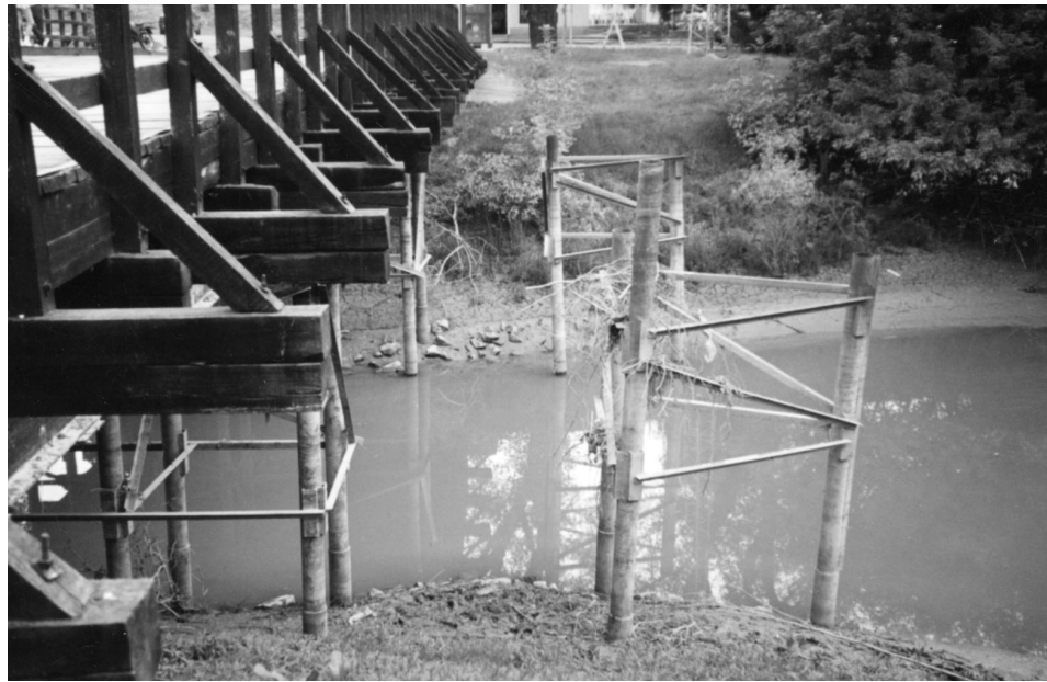
Figure 5.14 Sacrificial piles upstream of a bridge
