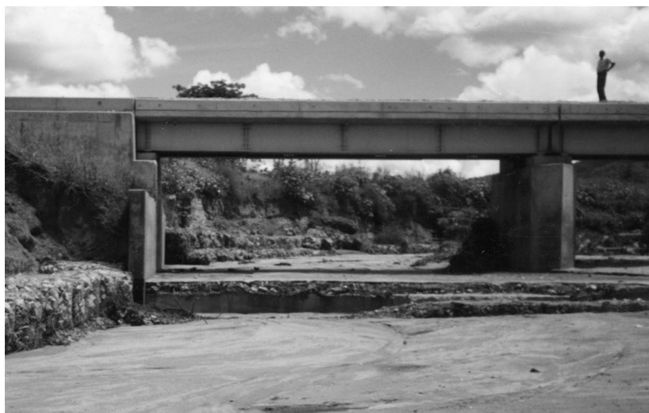
Figure 5.8 Scour caused by turbulence downstream of a bridge. The provision of a solid invert to a bridge almost inevitably leads to scour downstream. The gabion wall on the left of the picture has been added as an emergency measure to stabilise the bank
