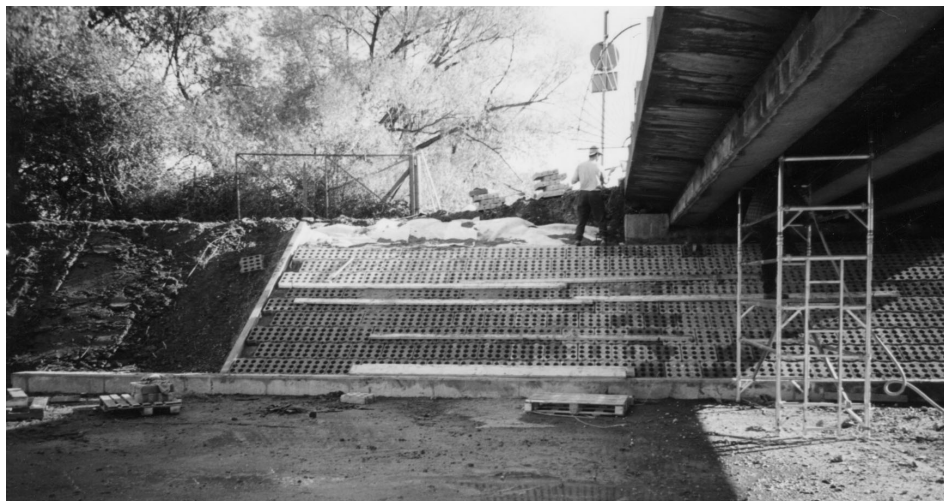
Figure 5.26 Interlocking concrete block protection to bridge (photograph courtesy of the Environment Agency)
