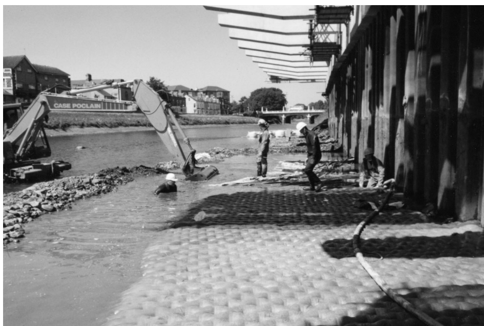
Grout-filled mattress protection to sheet-pile wall
