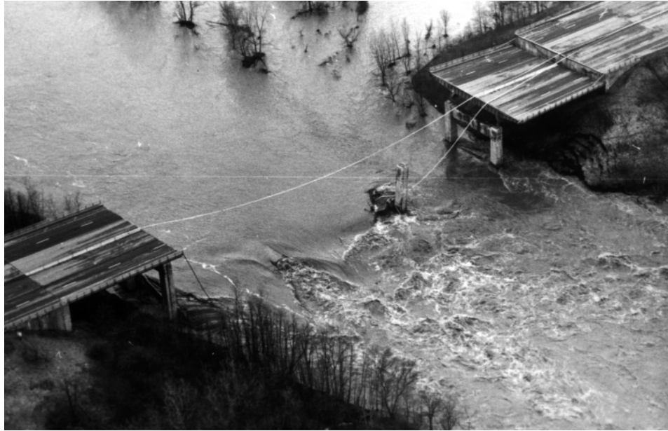
Figure A2.8 Schoharie Creek road bridge after collapse of second pier (photograph courtesy of Ayres Associates)
