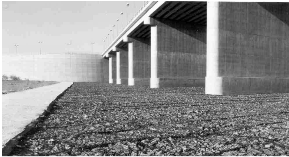
Gabion protection to bridge invert
