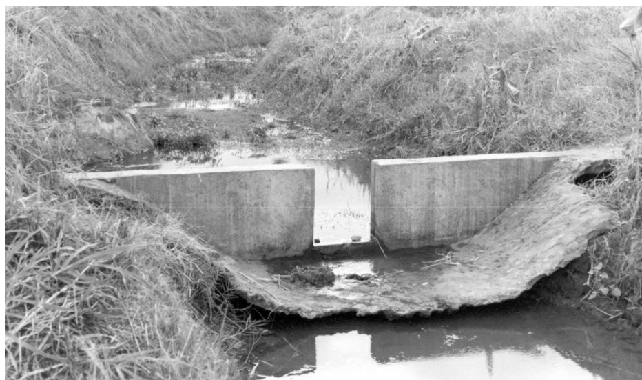
Figure 5.30 Scour downstream of a small structure, highlighting the problem with an inflexible concrete apron
