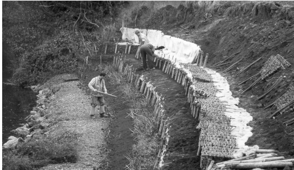
Figure 5.28 Construction of rock armour and willow faggoting repair to eroded river bank (photograph courtesy of Jeremy Benn Associates)
