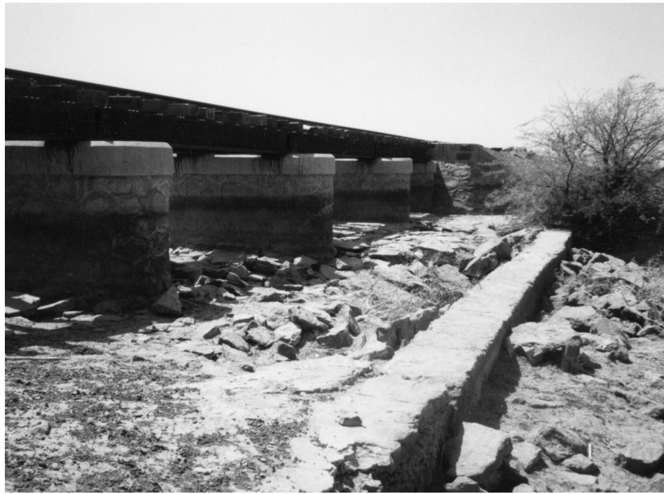
Figure 5.12 Bed control using a downstream sill. Note that poor construction has led to failure of the pitched stone apron, and that scour downstream of the sill – if left unchecked – could undermine the sill
