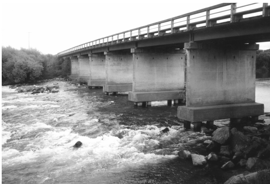
Figure A2.7 Oreti River road bridge (photograph courtesy of Stephen Coleman)
