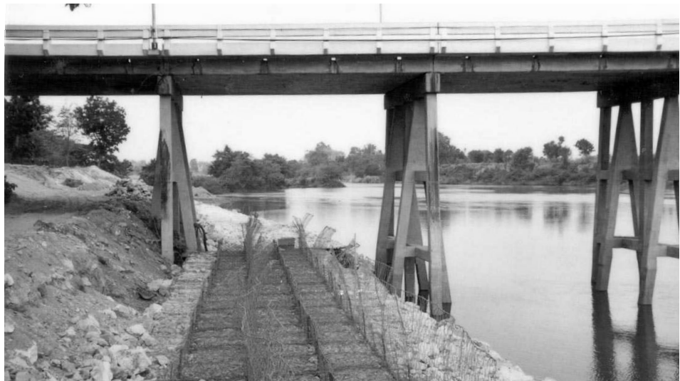
Gabion protection to bridge abutments
