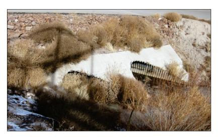
Figure 5.20. Slope paving around a mitered inlet.
