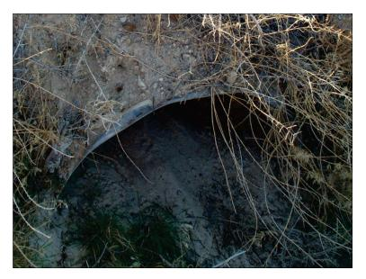
Figure 5.12. Excessive sediment deposition in culvert.
