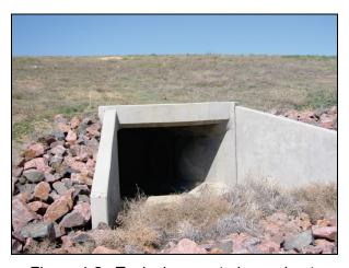
Figure 1.2. Typical concrete box culvert.
