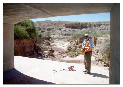
Figure 5.11. Stream degradation downstream of culvert outlet (from Utah DOT).
