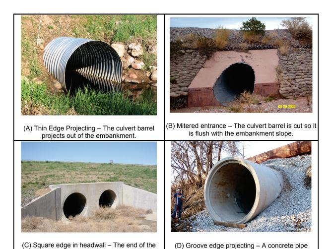
Figure 3.2. Typical inlet configurations.
