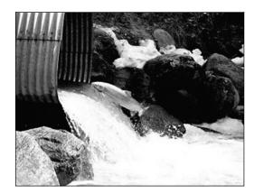
Figure 4.2. Jump and velocity barrier.
