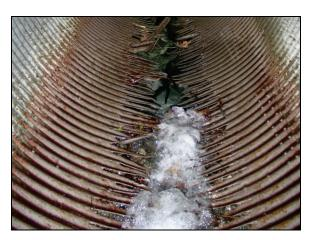
Figure 2.12b. Corrosion issues in a culvert.
