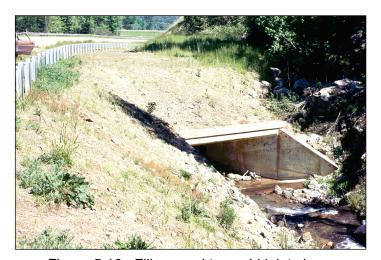
Figure 5.16. Fill warped to avoid inlet skew.
