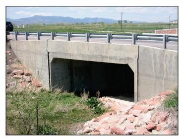
Figure 1.6. Concrete box culvert.
