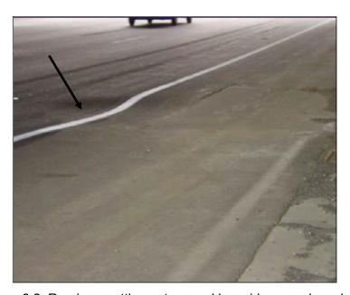
Figure 6.2. Roadway settlement caused by voids around a culvert.
