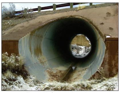
Figure 1.20. Structural plate culvert.
