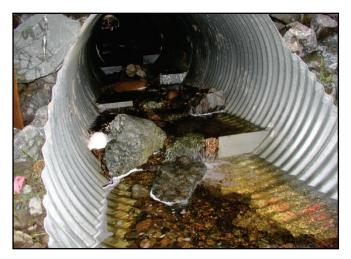
Figure 5.6. Alternating baffles.
