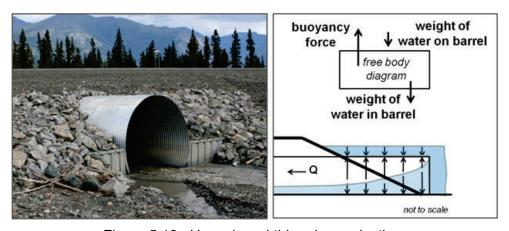
Figure 5.19. Unanchored thin edge projecting.
