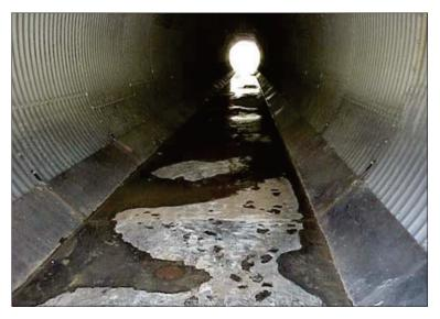
Figure 6.18. Invert repair of CMP using steel plating.
