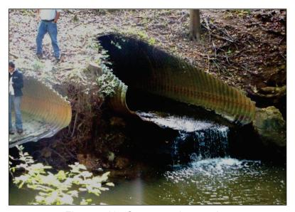
Figure 5.10. Scour at culvert outlet.
