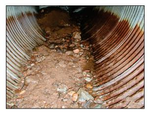
Figure 2.12a. Abrasion issues in a culvert.
