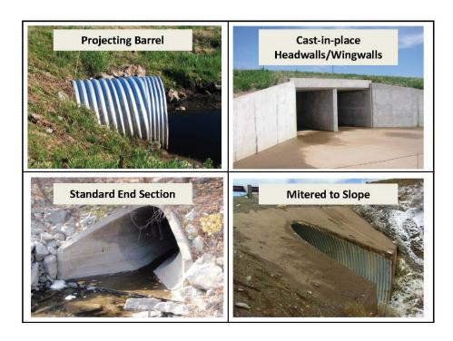
Figure 1.8. Four standard inlet types.
