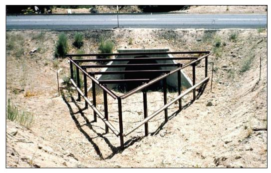
Figure 2.6. Steel rail debris deflector (looking downstream).
