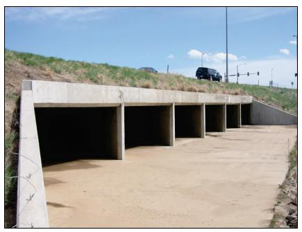
Figure 1.21. Multi-cell box culvert.
