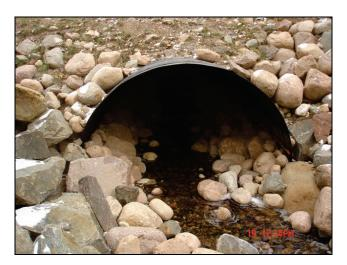
Figure 1.12. Embedded culvert (from WI DOT).
