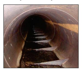
Figure 5.7. Angled baffles (from FishXing Users Manual).
