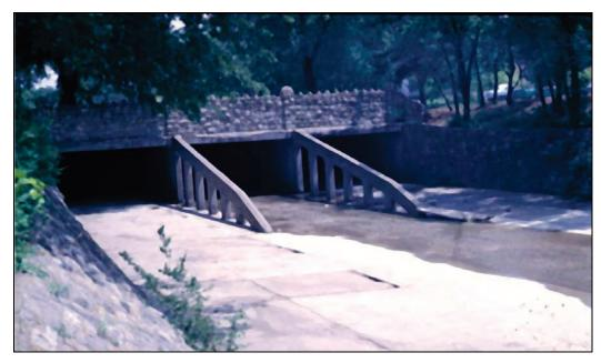
Figure 2.8. Concrete debris fins with sloping leading edge as extension of culvert walls.
