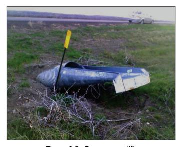
Figure 6.5. Buoyancy uplift.
