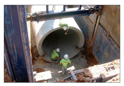
Figure 6.10. Open-trench excavation with shoring.
