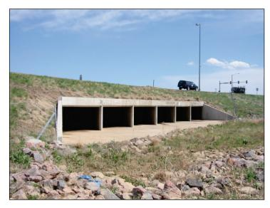
Figure 5.17. Multiple barrel box culvert.
