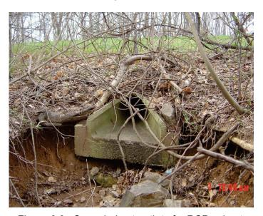
Figure 6.8. Scour hole at outlet of a RCP culvert.
