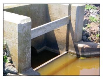
Figure 5.1. Culvert as outflow control device.
