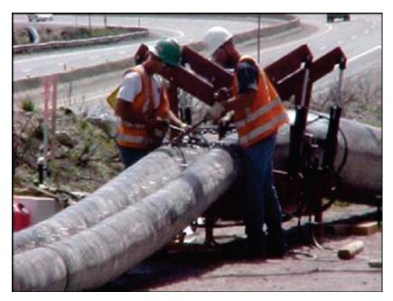
Figure 6.15. Deformed-reformed liner installation.
