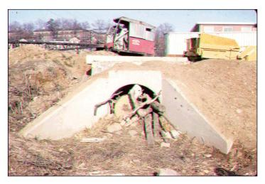
Figure 6.3. Severe debris blockage.
