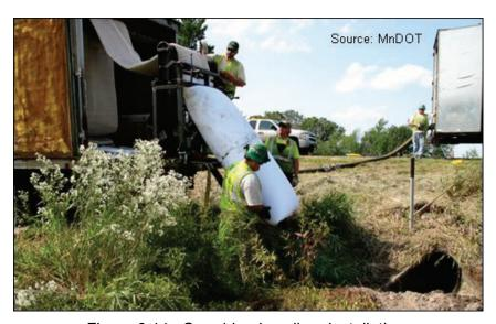
Figure 6.14. Cured-in-place liner installation.
