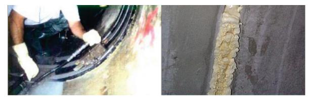
Figure 6.17. Joint repair using gaskets and joint sealing via person-entry.
