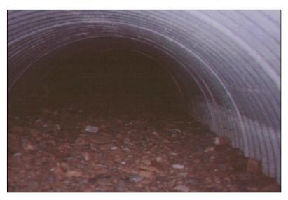
Figure 6.4. Barrel filled with sediment up to half its rise.
