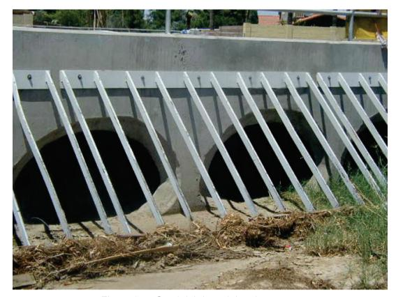
Figure 2.7. Steel debris rack in urban area.
