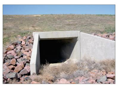
Figure 5.9. Inlet protection based on headwall, wingwalls and riprap.
