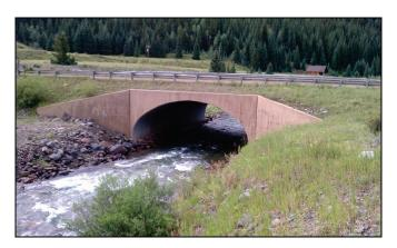
Figure 1.11. Open-bottom culvert.
