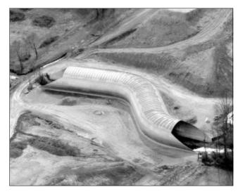
Figure 5.3. Culvert with a horizontal bend (Contech).
