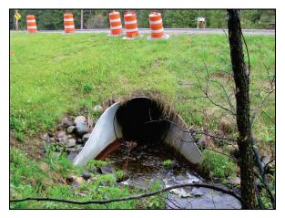
Figure 1.1. Typical small corrugated metal pipe culvert (from WI DOT).
