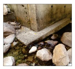
Figure 6.9. Exposed spread footing in an open-bottom culvert.
