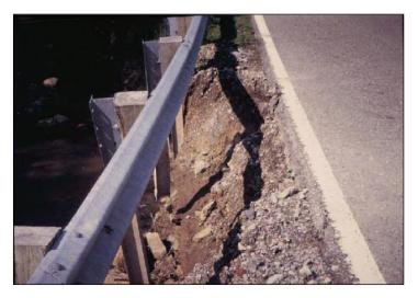
Figure 6.7. Erosion damage to downstream embankment slope from overtopping.
