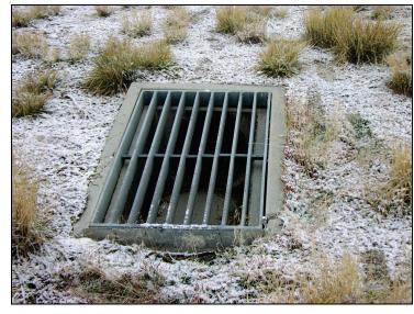
Figure 2.11. Traversable safety grate with proper open area between bars.
