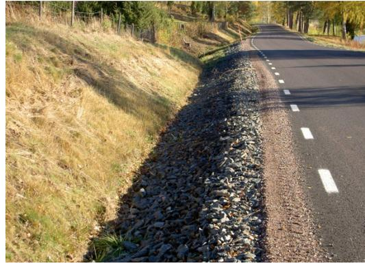
**Fig.1. Surface drainage system, photo: VTI**
