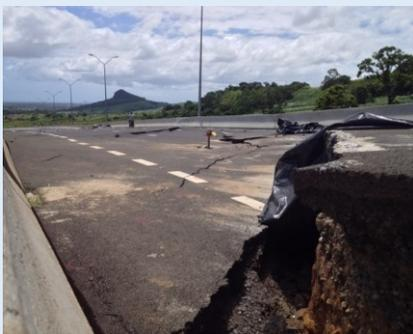
The Terre Rouge-Verdun road was damaged due to landslide after a heavy downpour.
