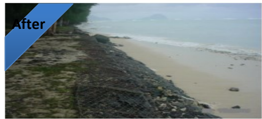
Beach protection works at Flic en Flac public beach
