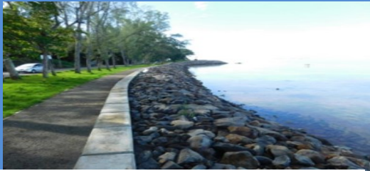
Rock revetment for shoreline protection at Baie-du-Cap
