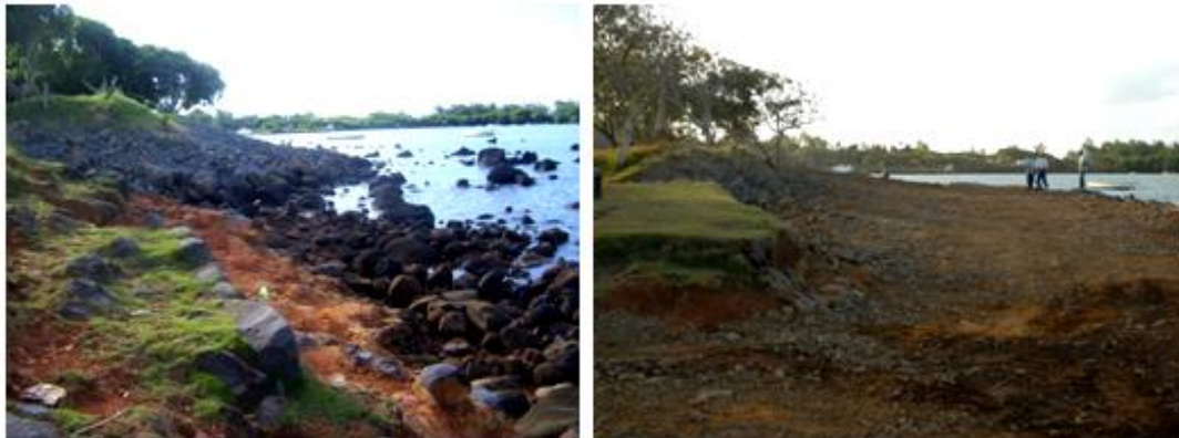
Figure ES 5(a) - Beach eroded (left) and 59(b) being rehabilitated (right). (Courtesy photo: ADD)
