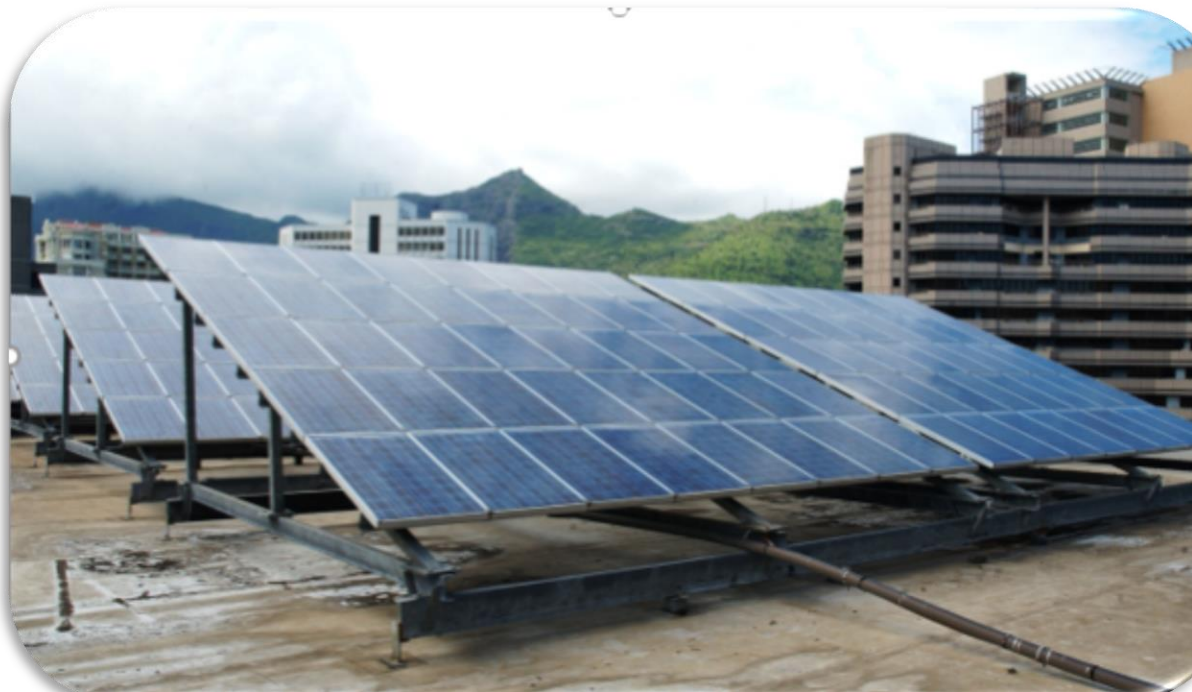
Figure 4.1: Photovoltaic solar panel on rooftop, an incentive to reduce dependency on fossil fuel. (Courtesy: GIS)
